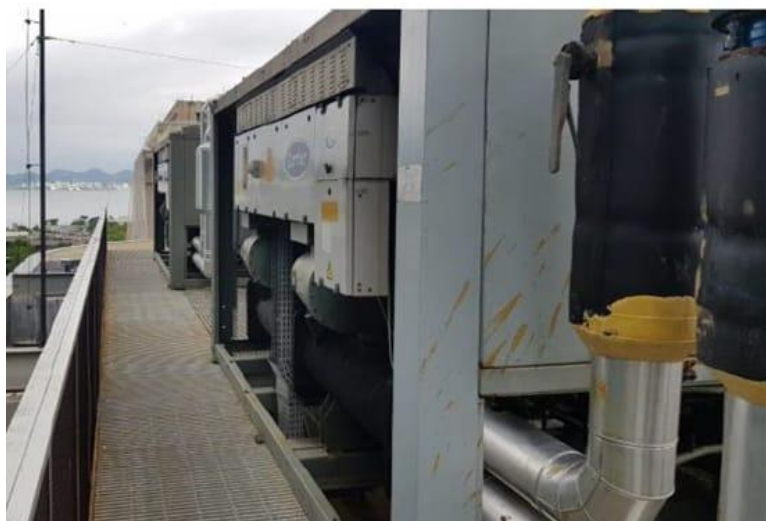
Chiller Parafuso CARRIER Mod. 30GX
